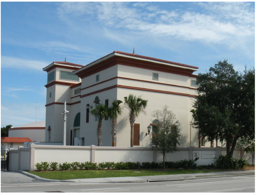
Town of Jupiter Water Utility Plant, 17403 Central Boulevard, Jupiter, Florida
